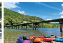
Takase Submersible Bridge
