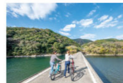
Katsuma Submersible Bridge
